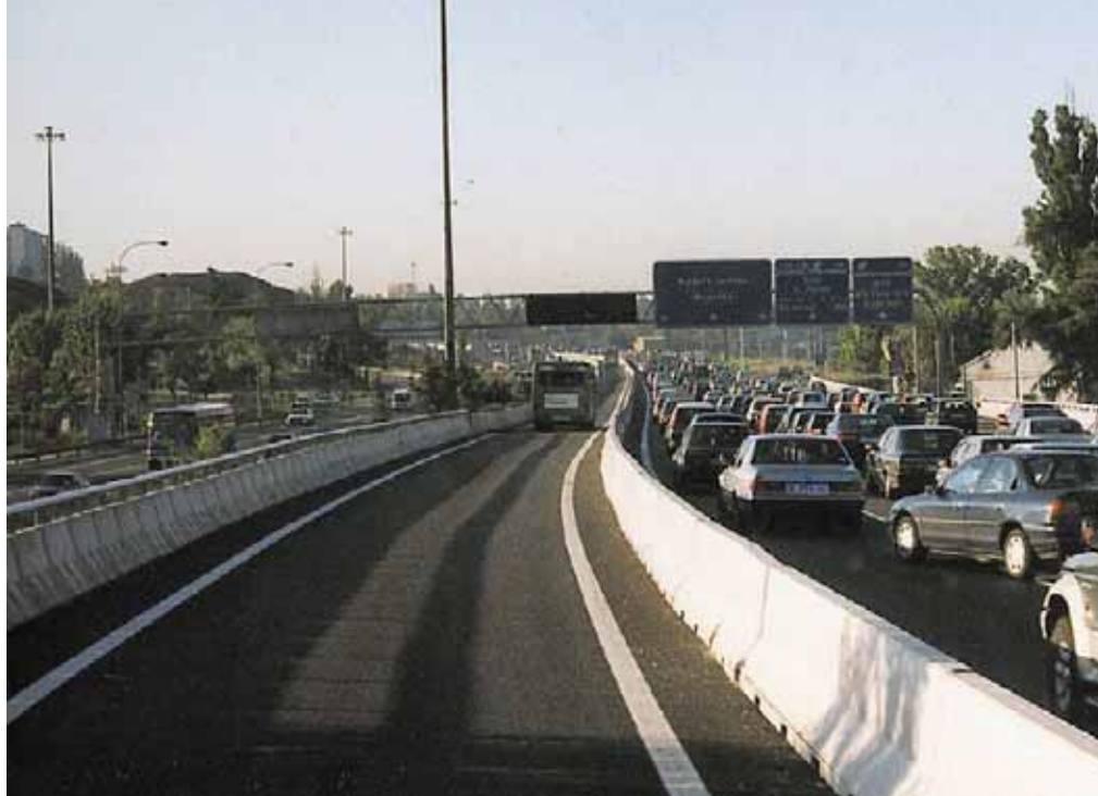
Carril Bus-Vao de la A6 / The Bus-HOV lane on the A6 road
