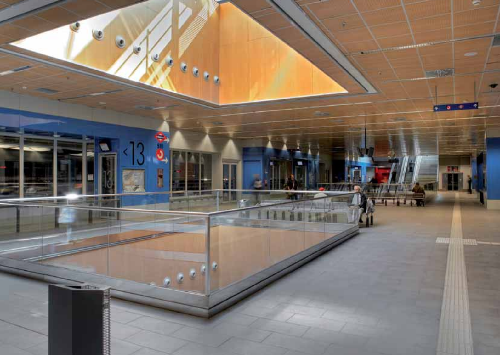
Entrada de luz natural a través de lucernarios Entry of natural light through the light wells
