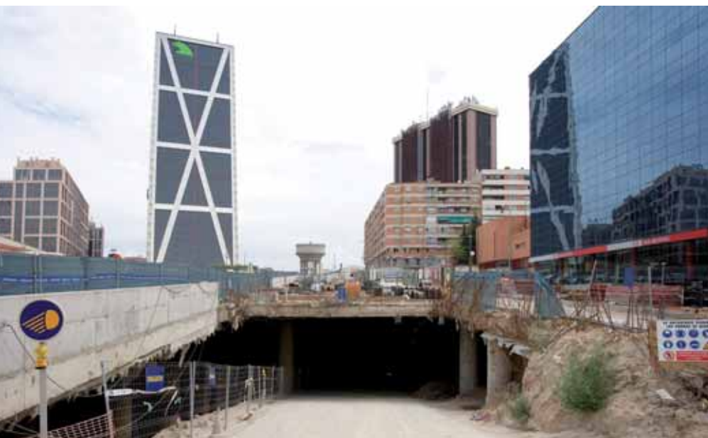
Plaza de Castilla transport interchange station
