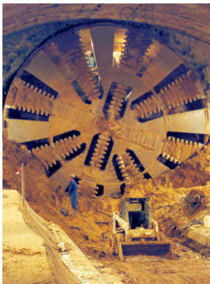
Tunnelling machine entering a Metro station
