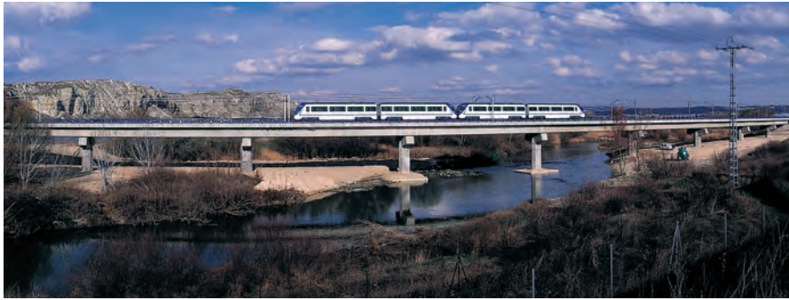
Line 9 on its way over the River Jarama bridge
