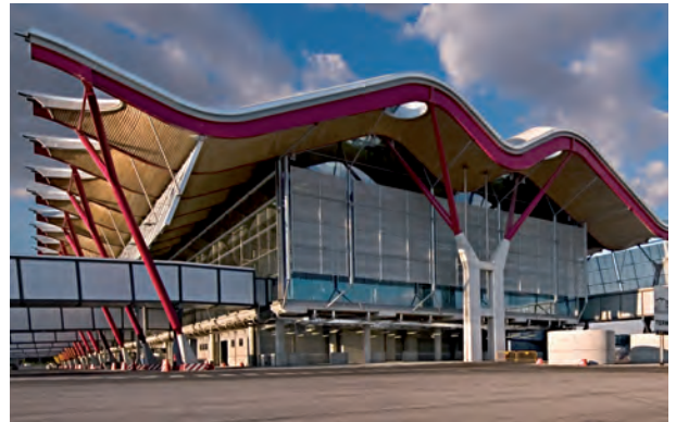
Madrid-Barajas Airport. Rogers and Lamela
