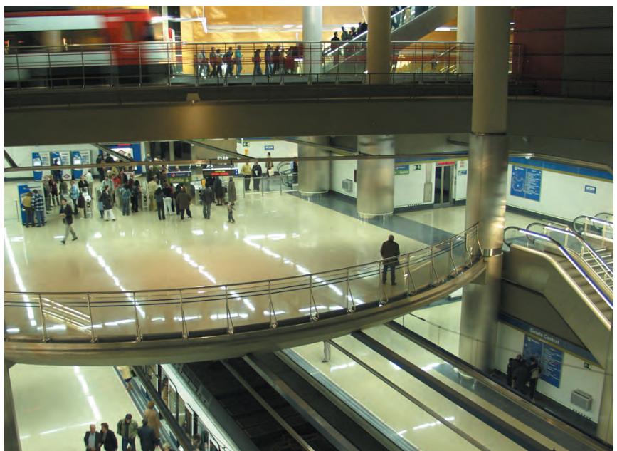
Getafe Central Station on the day it opened
