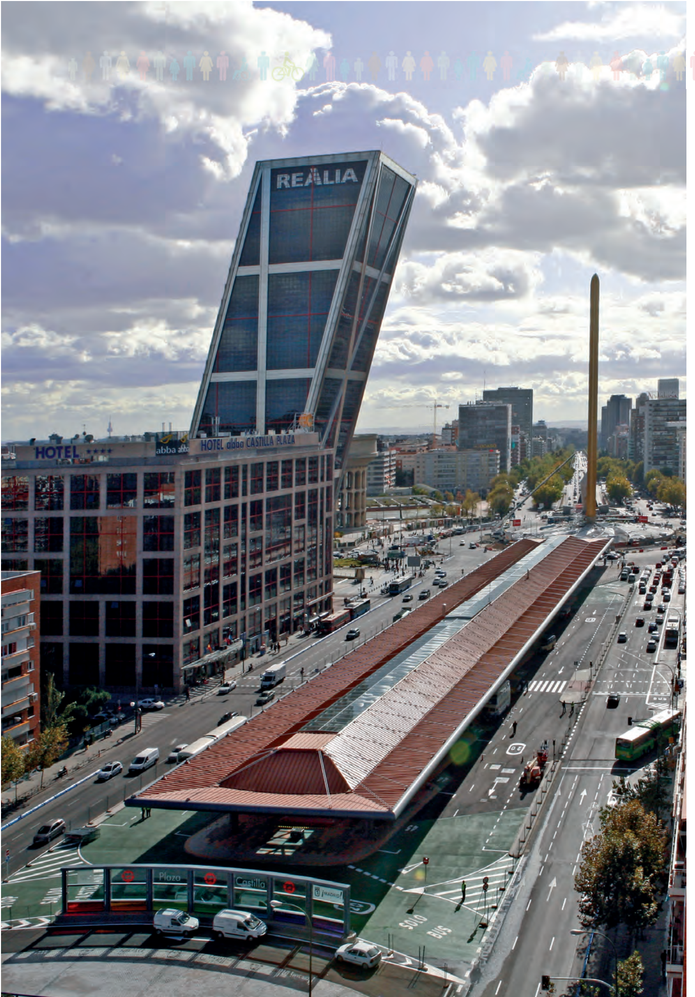
Surface interchanger at Plaza de Castilla
