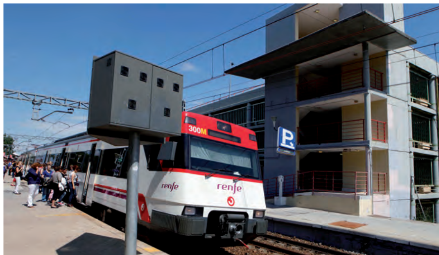
Pay park-and-ride car park at Majadahonda station
