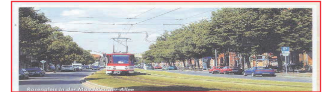
The new 'green' tram tracks in Erfurt.
