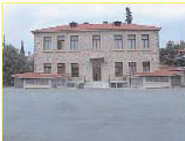
BEFORE: The site for the Panorama car park.
