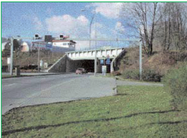
The new section of the Brno ring road.
