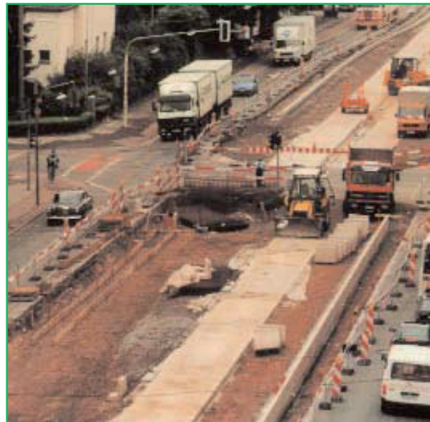
The Saarbahn under construction.
